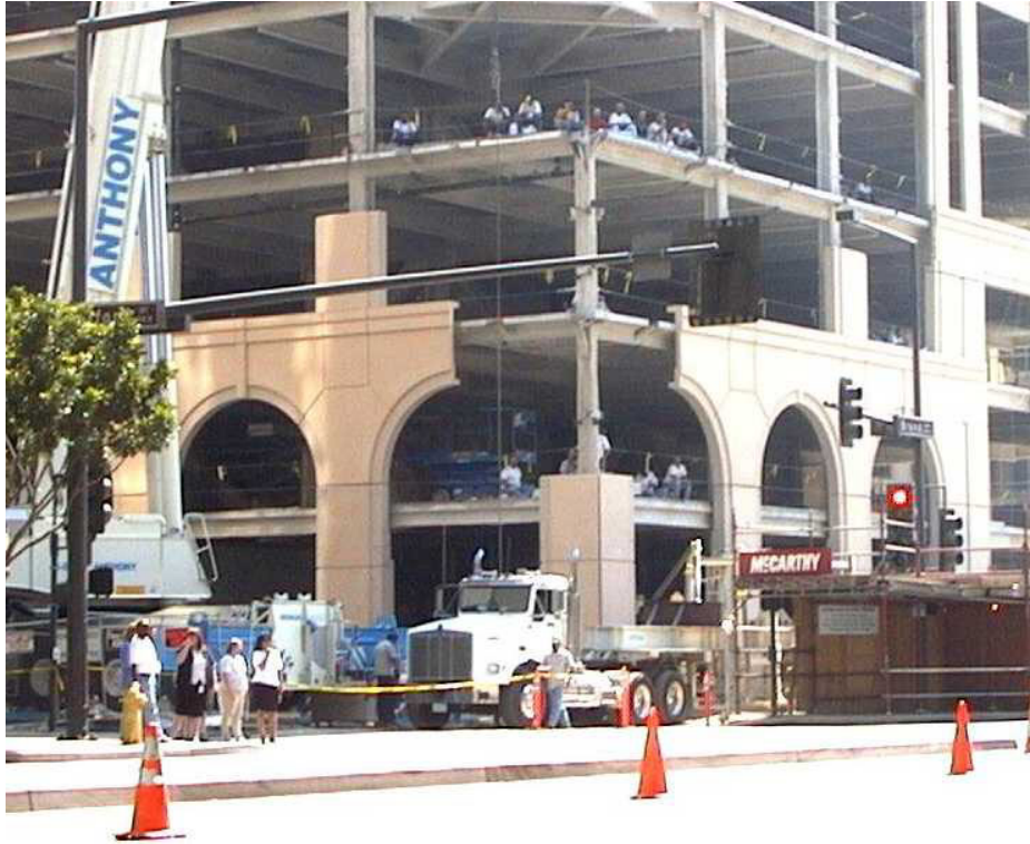
(a) Precast cladding.
